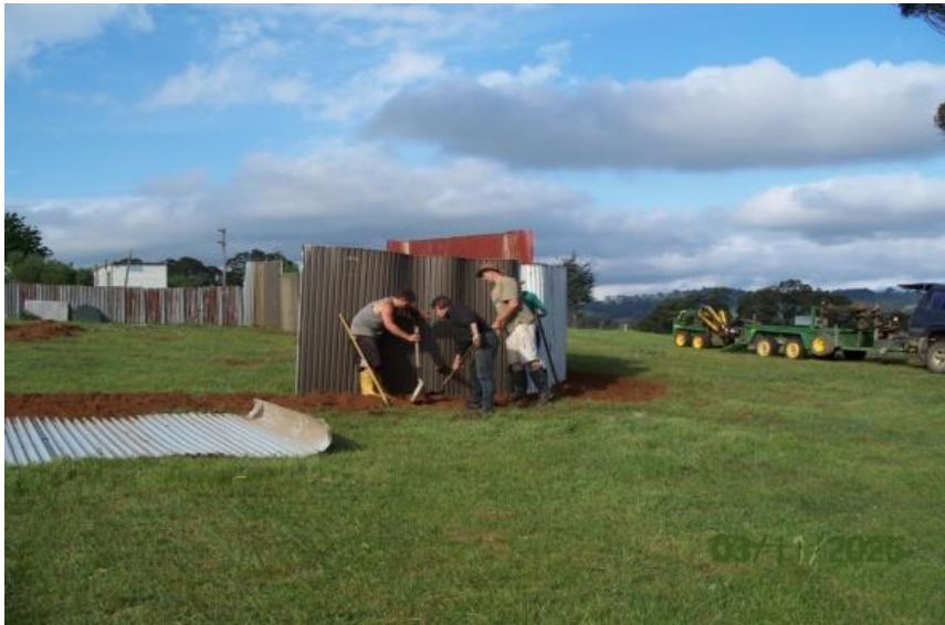
STARTING TO BUILD A NEW COMPOUND
