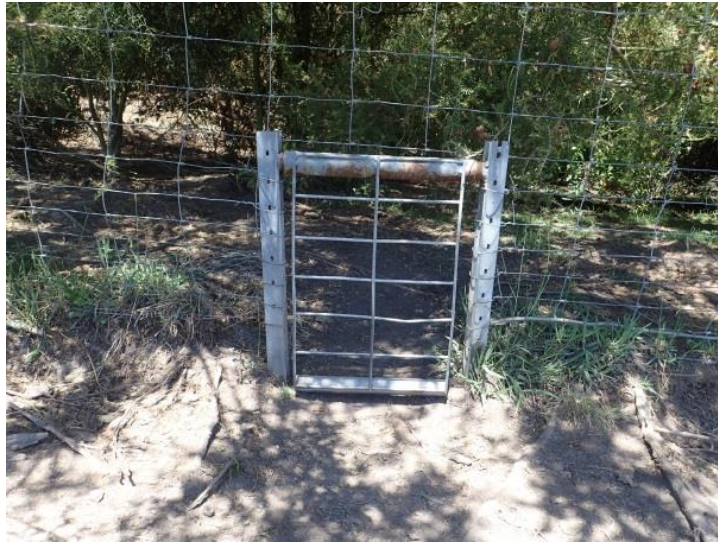
Light gate with hollow base bar
